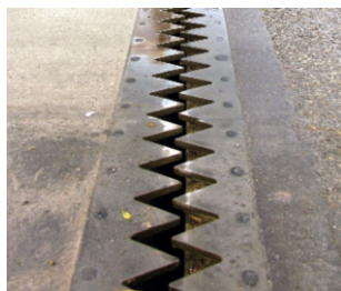
Figure 12.6: Expansion margin in a bridge.
